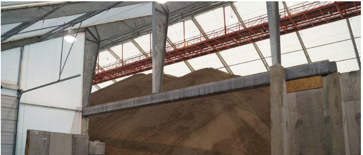
Figure VII: Jack beams allow for exceptionally wide side wall openings
