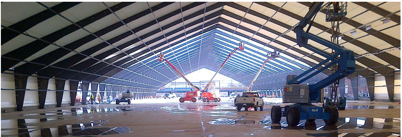
Figure VIII: Fabric panel installation
