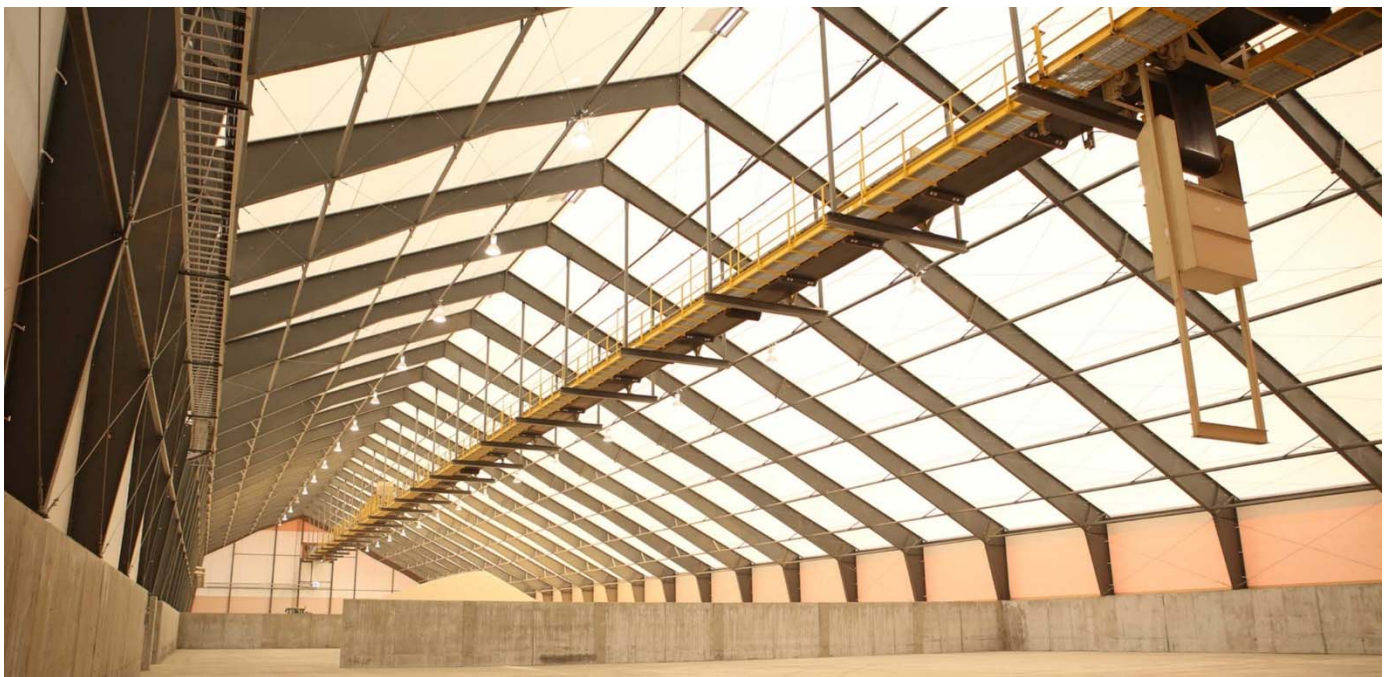
Figure VI: Fabric building interior with steel I-beam frame
